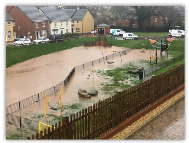
The probable cause of this is a blockage of the orifice plate by the quantity of silt washing off the surrounding fields and into Sluts Brook.
