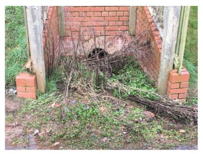
Alongside this, the rubble from when the headwall drainage outlets were originally built (4 years ago) has never been cleared of bricks and builders rubbish and this remains a problem, inhibiting rain water drainage.
