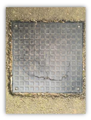
DWH assured us, last summer (2020), that an audit would be undertaken across site to ascertain which drain covers had been incorrectly installed and that these would be replaced with correctly specified ones. However, this hasn't happened and many of the existing drain covers remain contrary to building regulations, whilst also representing a health and safety issue.
