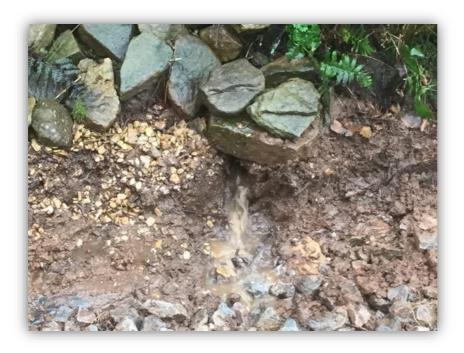
Although DWH have now carried out remedial works at plot 41, digging out the back-filled pipe and installing a gravel filter drain along part of it, these works are unlikely to be fully effective due to the silting up of the underground culvert detailed below, and the sheer volume of run-off at that corner of the field.
